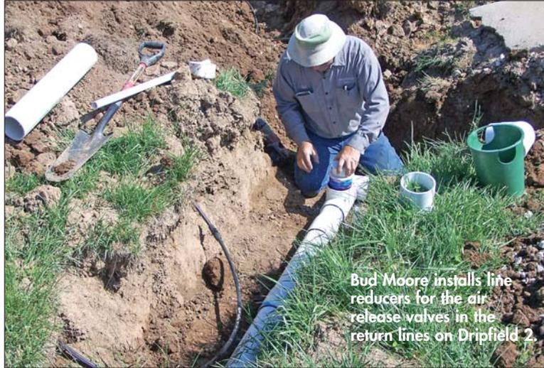
Bud Moore installs line reducers for the air release valves in the return lines on Dripfield 2.
