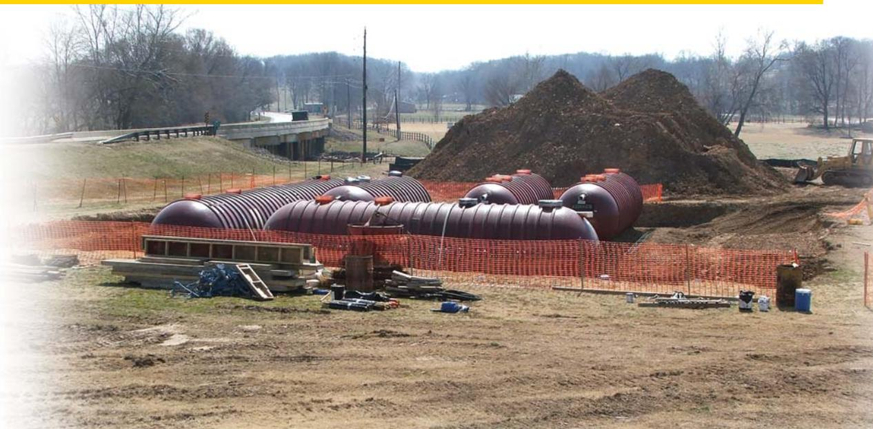
Fiberglass tanks in the process of installation at the treatment plant site. (Photos courtesy of Aqua Tech Systems LLC)
